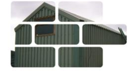
The metal profile sheet is a strong lightweight product made from flat coated steel that is molded into a range of trapezoidal/box, tile or corrugated profile shapes. These are base coated, galvanised and then top coated with polyester paint, PVC plastisol or other finish in a wide range of colours to resist corrosion. Barge, fascia, corner and ridge boards are made in the same way. They are all malleable to suit most architectural designs.
