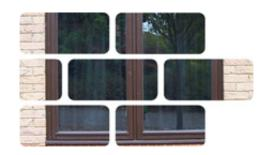
Timber windows are made in various sizes, types and arrangements depending on the specification required. They are of varying quality, from softwood small profile windows to more desired hardwood windows or specialist display windows. Most windows are mass produced, whereas some are made-to-measure to suit a particular architectural finish. All windows will incorporate glass or glazed units and a range of fixtures.
